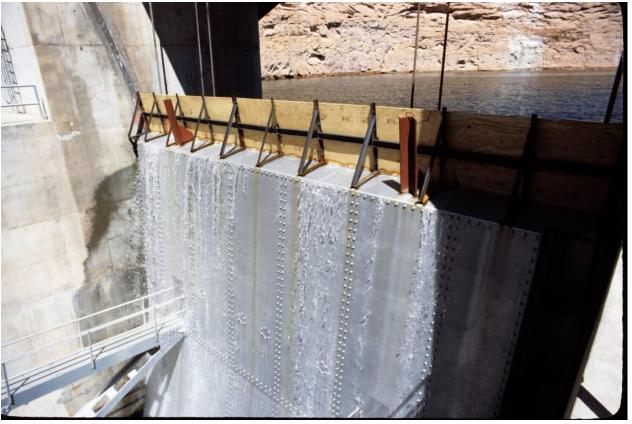
Water got so high at Glen Canyon Dam that a plywood flashboard was improvised to prevent overtopping of the spillway gate.
