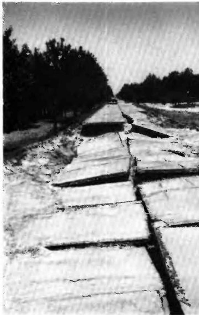
Figure 30. --U. S. 190 near Kinder, La., damaged by flood on Calcasieu River. Crest of flood covered road about 2 feet.
