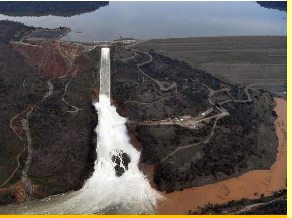
What can be seen is the result of the massive collapse (pictured) when 100,000 cubic feet of water per second was rushing down the spillway
