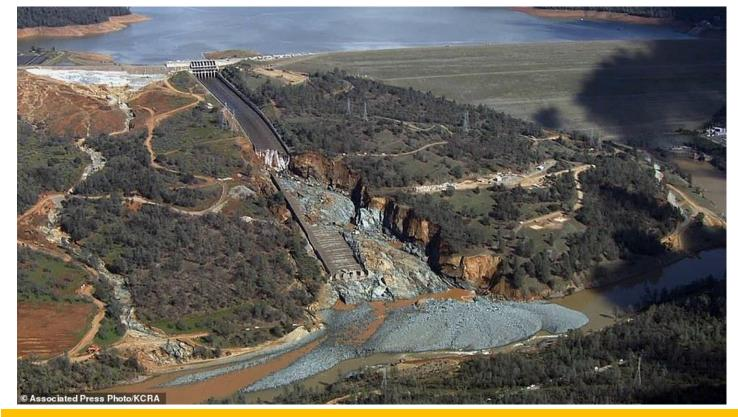
A bird's eye view taken on Monday shows the massive pile of grey rubble that has settled at the bottom of the spillway. Because of the damage, the water flow is not fast enough to clear any of the rubble when it reaches the bottom
