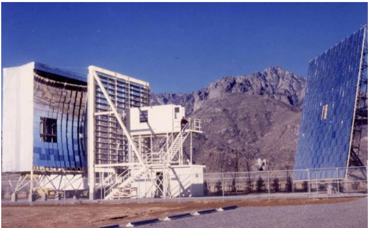
Figure 2. Picture of WSMR Solar Furnace with Organ mountains in the background.
