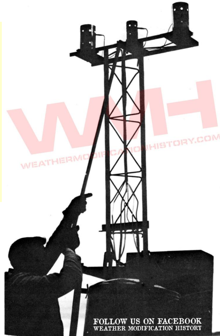
A silver iodide generator, a prime tool of the weather modifier's trade, is raised vertically by EG&G Company employee at Fort Lewis College.
