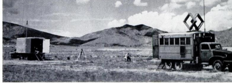
Radar truck tracks cloud formations and radio direction-finding truck records lightning 1000 miles away
