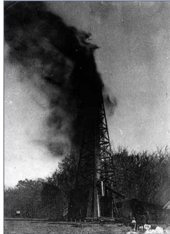
First 30 years of drilling was done by inexpensive cable tools rigs with wooden derricks.
