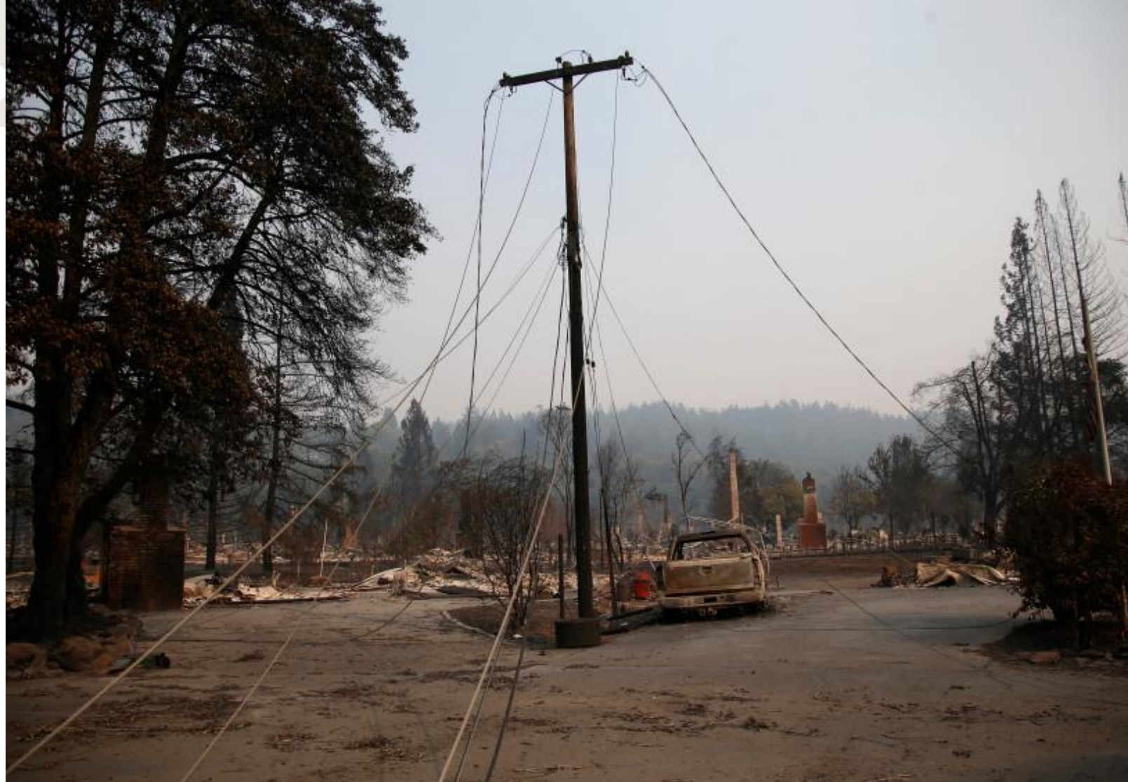
Fallen electrical lines on Parker Hill Road in Santa Rosa on Tuesday. (Nhat V. Meyer/Bay Area News Group)
