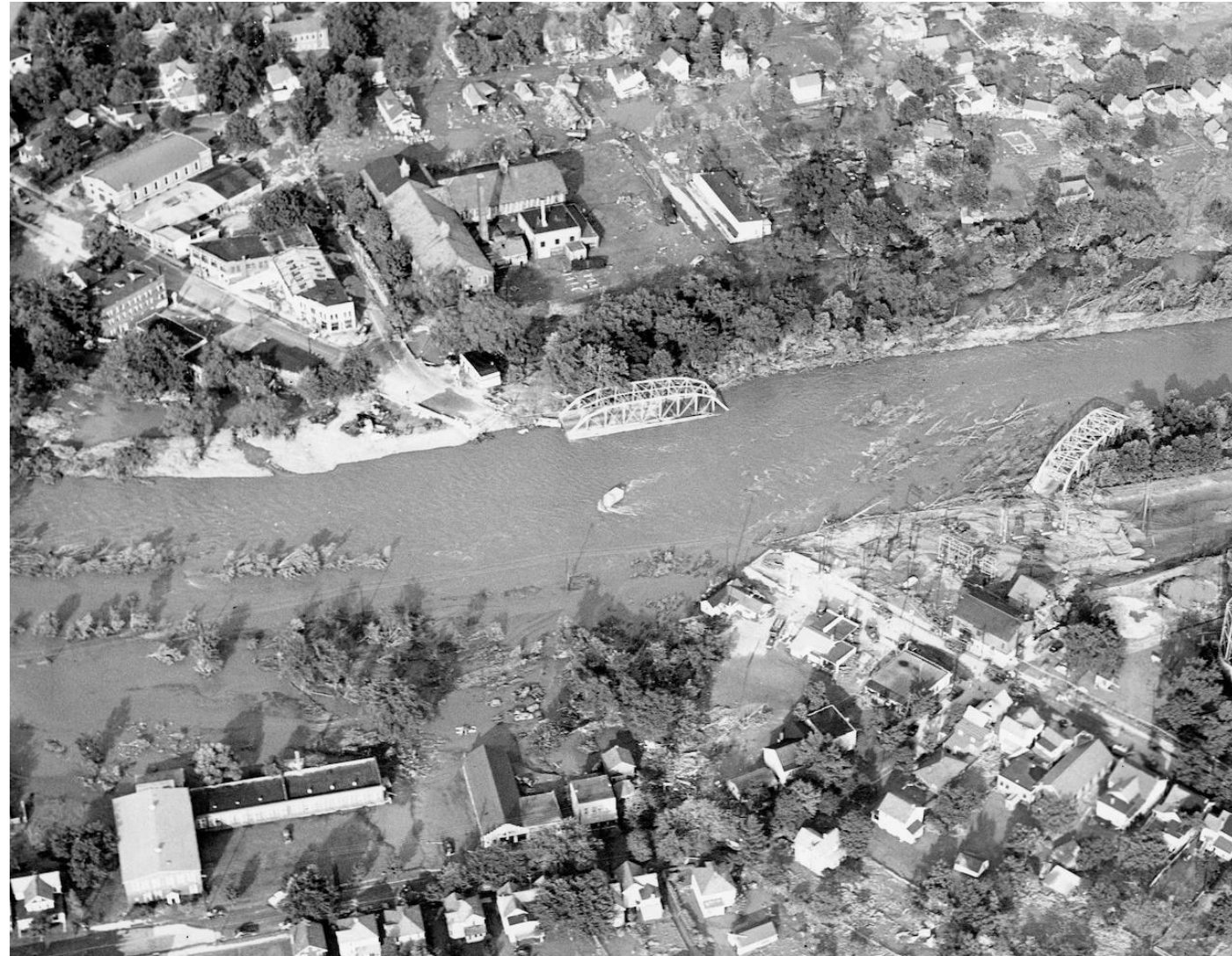
A bridge is washed away as a result of flooding from Hurricane Diane in August 1955. Location unknown. (The Evening News)
