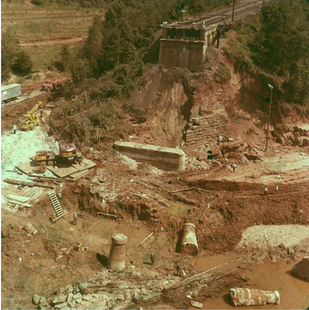
Close up view of the North abutment of the bridge.
