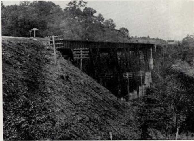
Second bridge over the Tye was completed in 1915 as a part of the double-tracking of Southern between Washington and Atlanta.
