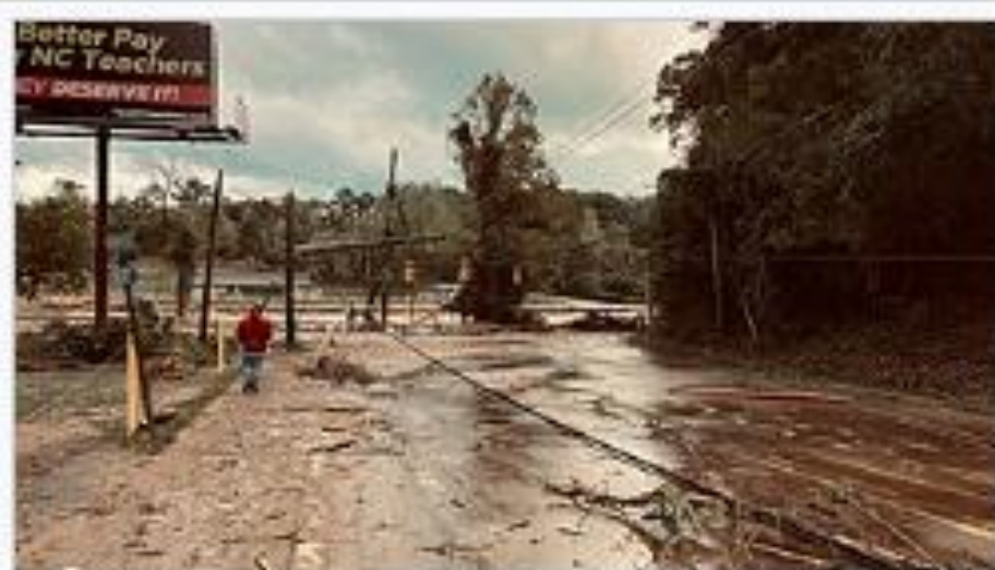
Devastation in Asheville, North Carolina – at the intersection of Swannanoa River Road (NC-81) and Azalea Road – caused by Hurricane Helene
