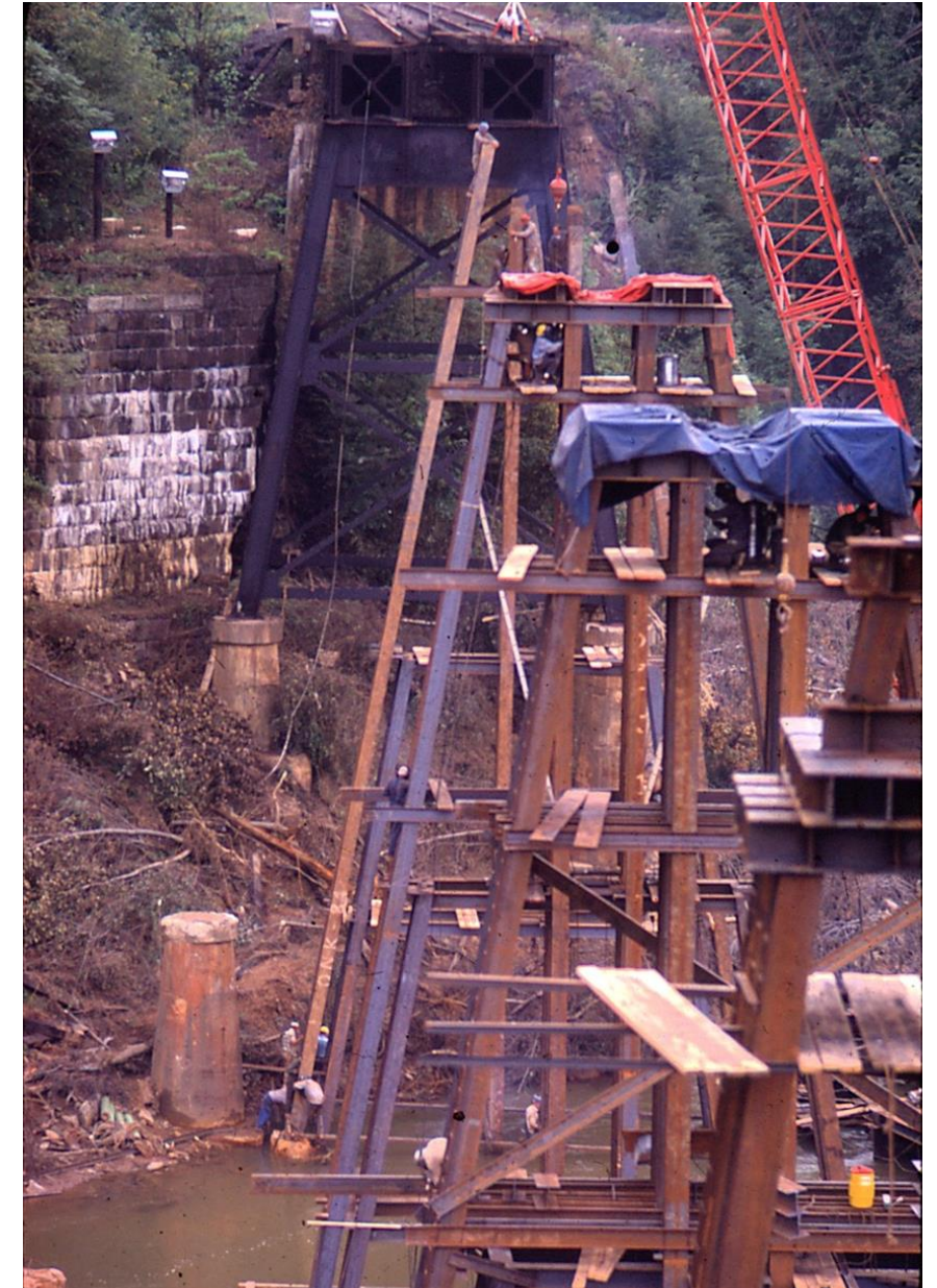
Tower bents under construction. Notice that caps are in place for the bent in the right foreground ready eventually to receive spans
