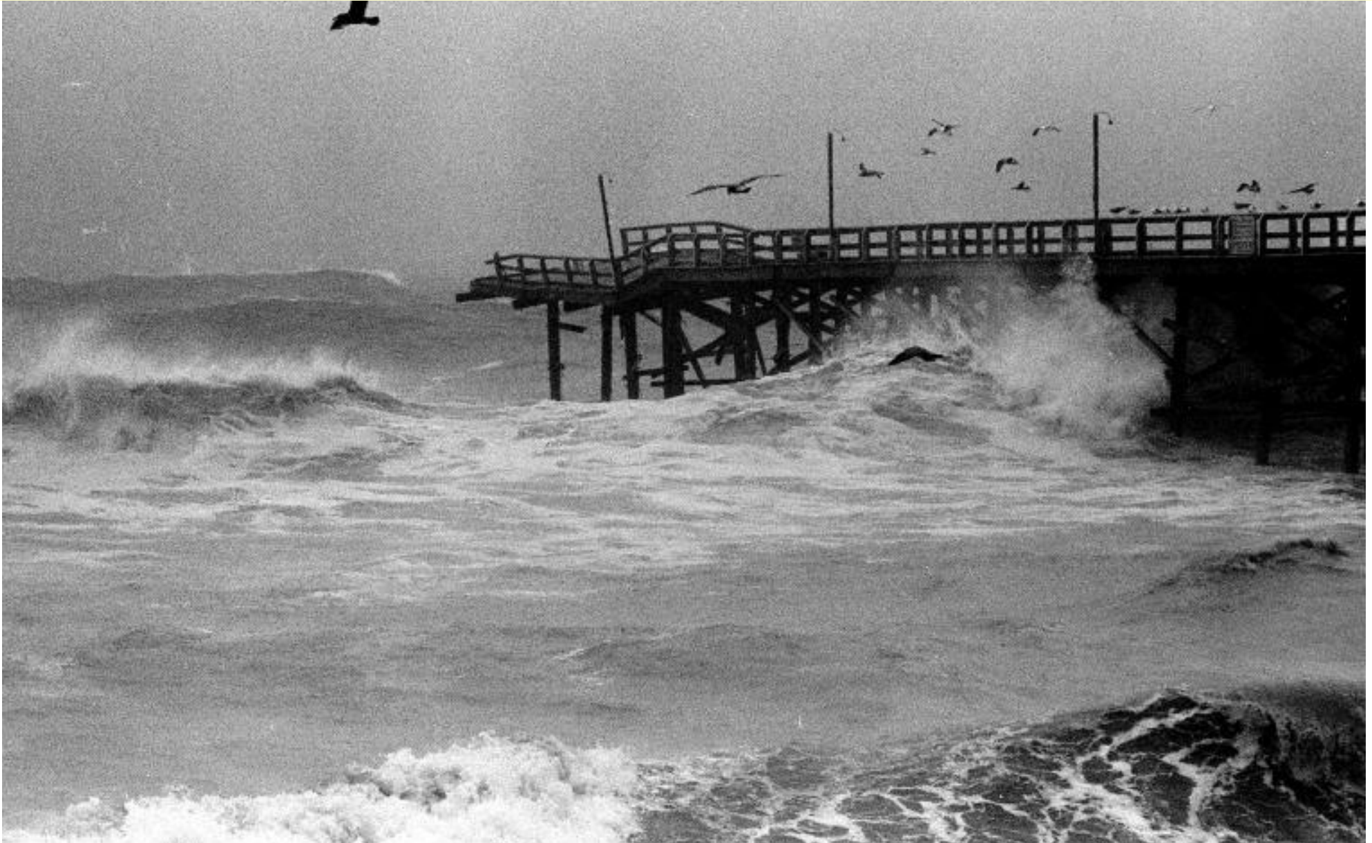
The landmark Crystal Pier off Pacific Beach collapses under the force of surging waves during an El Niño storm in San Diego on 27 Jan 1983.
